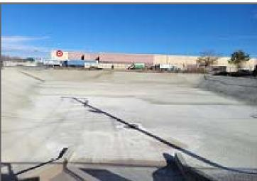
D18 City\_Quad MAP\_KEY NE Year\_Built 2022 X:\MD\SHARE\MD-Storm\Ponds-Trash Racks-cat\2-TRASH RAC FIBER REINIFORCED SHOTCRETE ( 3" FOR THE BOTTOM, 2" FOR THE SIDES) NOTES SWQ SIZE 1656 SY LINING cost \$205,500 PROJECT\_NO 52809 NUMBER 191
