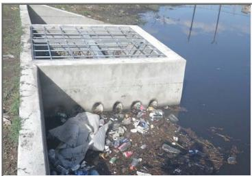
City\_Quad MAP\_KEY K14 SW Year\_Built 2021 X:\MD\SHARE\MD-Storm\Ponds-Trash Racks-cat\TRASH\_RACKS INSIDE SOUTH BROADWAY POND NOTES 8' X 8' X 4 1/2' WITH 6" DIA TUBES 12" OC COVERED WITH 2" X SWQ SIZE cost \$122,000 2"WIRE MESH PROJECT\_NO 797200, 802614 NUMBER 16
